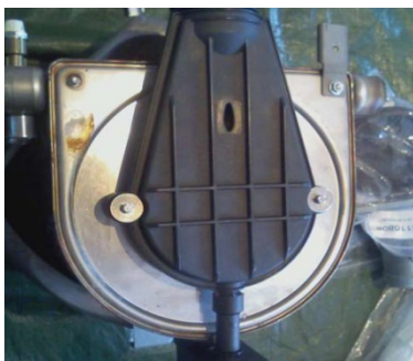
Figure 4 Black composite plastic flue/condensate connector attached to the rear of the heat exchanger (Photograph shows the view from the rear of the boiler)
